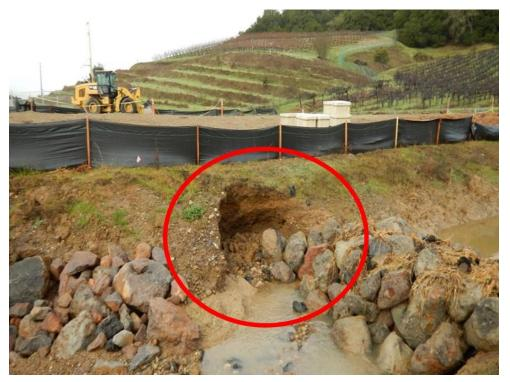
Figure 17. Lack of erosion and sediment controls in this inactive area resulted in stream bank failure that led to sediment deposition within Foss Creek
