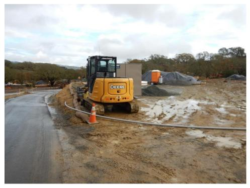
Figure 9. Disturbed soil where resort area was under active construction; lack of effective erosion or sediment control BMPs.
