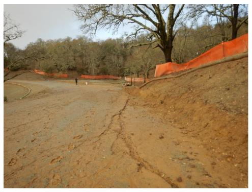
Figure 10. No linear sediment controls along the base of this roadside slope. Signs of gullying on the road.
