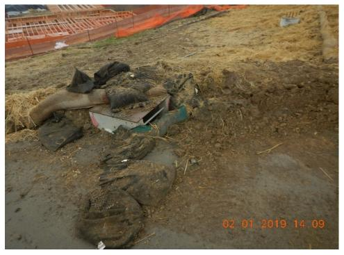
Figure 33. Sediment from the adjacent work area is overflowing onto the roadway and into the drain inlet.
