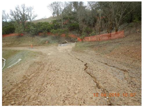
Figure 14. Road segment with no erosion and sediment control BMPs. Signs of gullying on the road.
