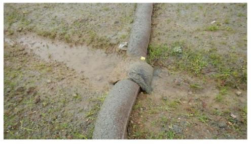
Figure 19. Ineffective soil cover contributing to erosion. The combination of BMPs for erosion, sediment, and turbidity controls on the Site was not adequate to prevent erosion and sedimentation.
