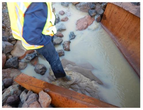
Figure 16. Significant sediment deposition within Foss Creek culvert inlet.
