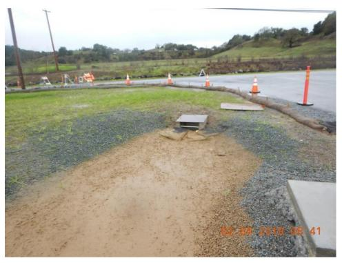
Figure 38. Downstream of Figure 37 above, sediment has overtopped the gravel bags and discharged sediment-laden runoff to the storm drain system that discharges to Foss Creek.
