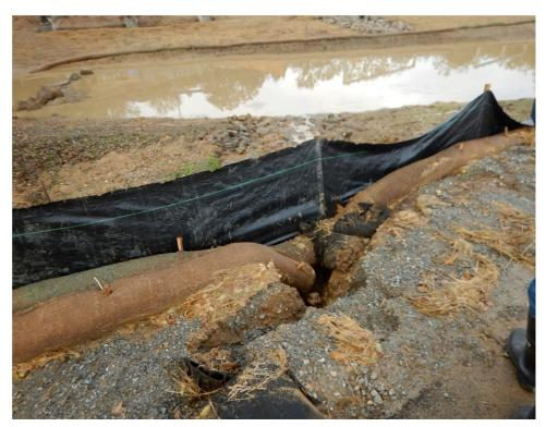
Figure 11. Erosional gully underneath wattle and silt fence; creek in the background.
