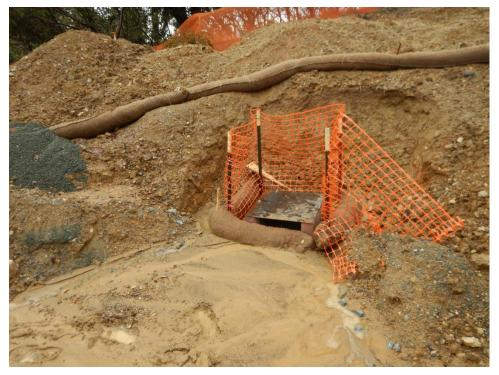
Figure 7. Sediment control BMPs inadequate to prevent erosion and overwhelmed by sediment deposition resulting from sediment-laden runoff.
