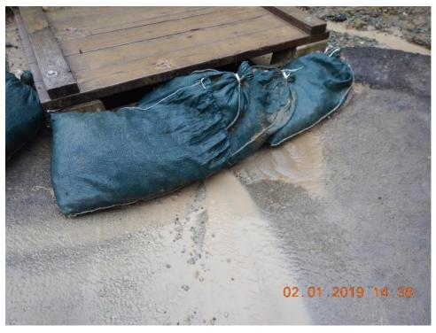
*Figure 35. This check dam is not correctly positioned to effectively capture or remove pollutants from storm water runoff.*
