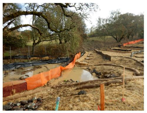
Figure 12. While several types of erosion and sediment controls are present at this location, the resort area lacked effective controls to prevent highly turbid runoff to the unnamed tributary (shown on left of photo) to Jordan Pond
