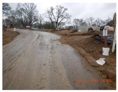
Figure 32. Sediment control BMPs observed do not effectively contain soil within the active construction area.
