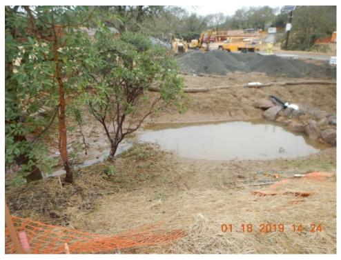
Figure 21. Uncovered stockpile near top of a stream/drainage channel bank. Creek in the foreground.
