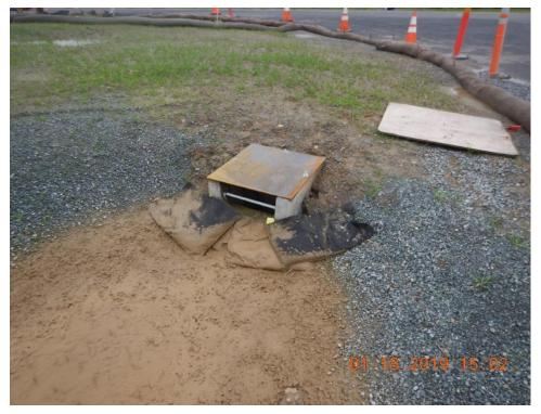
Figure 26. The sediment trap is inadequate and needs maintenance; sediment has overtopped the gravel bags and discharged sediment-laden runoff to the storm drain system that discharges to Foss Creek
