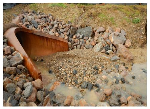
*Figure 18. Downstream from Figure 14, large sediment deposit within Foss Creek as a result of the slope failure along the creek bank.*
