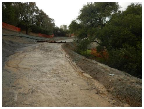
Figure 13. Road segment with adjacent unprotected slope and signs of uncontrolled runoff.
