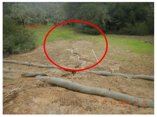
Figure 22. Sediment deposition beyond the undermined and overwhelmed BMPs; insufficient maintenance of erosion and sediment control BMPs.
