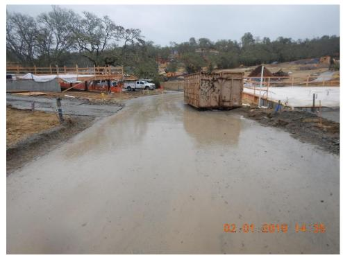
Figure 30. Mud on paved roads continues to result in discharges of sediment-laden runoff.
